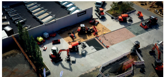
Model construction site at Coreum, Stockstadt a. R.
